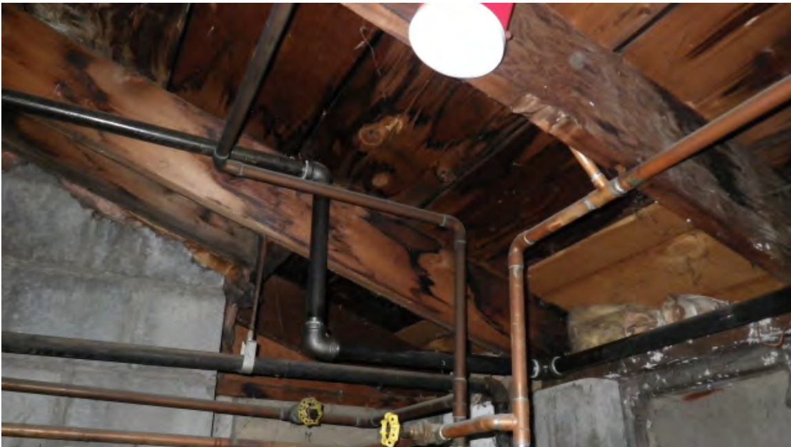
Photo 06 - Water-damaged roof framing at Fire Station boiler room
