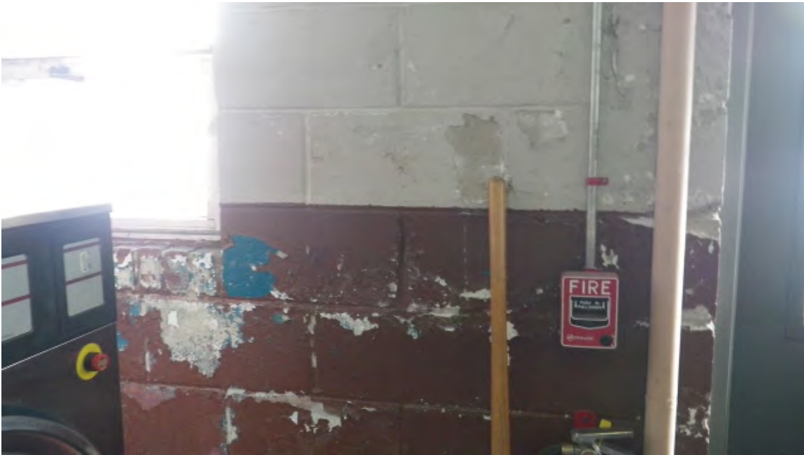
Photo 05 - Inside Fire Station. Note deteriorated block and mortar joints.
