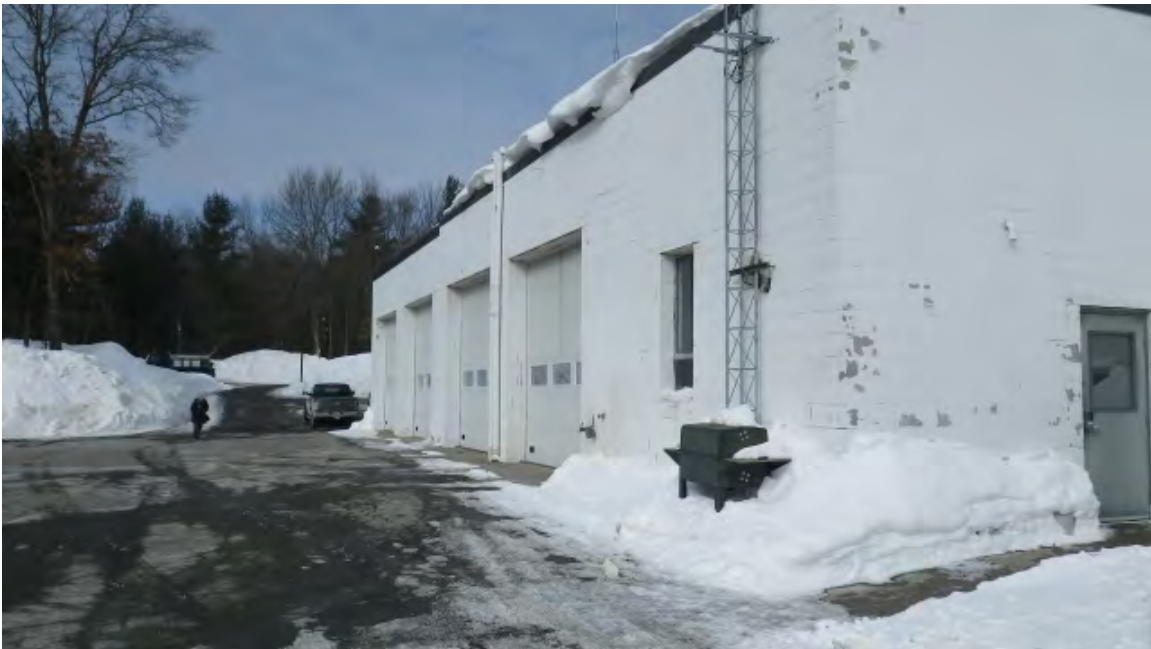
Photo 04 - Rear of Fire Station. Note deteriorated block and mortar joints.
