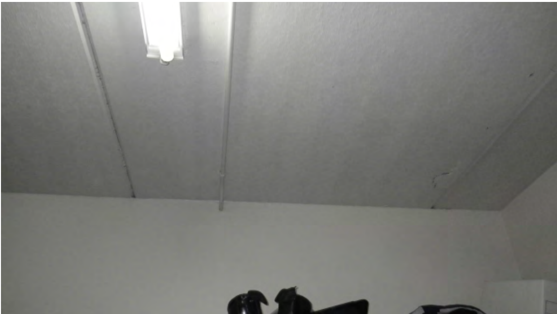
Photo 02 - First floor concrete planking at Police Station
