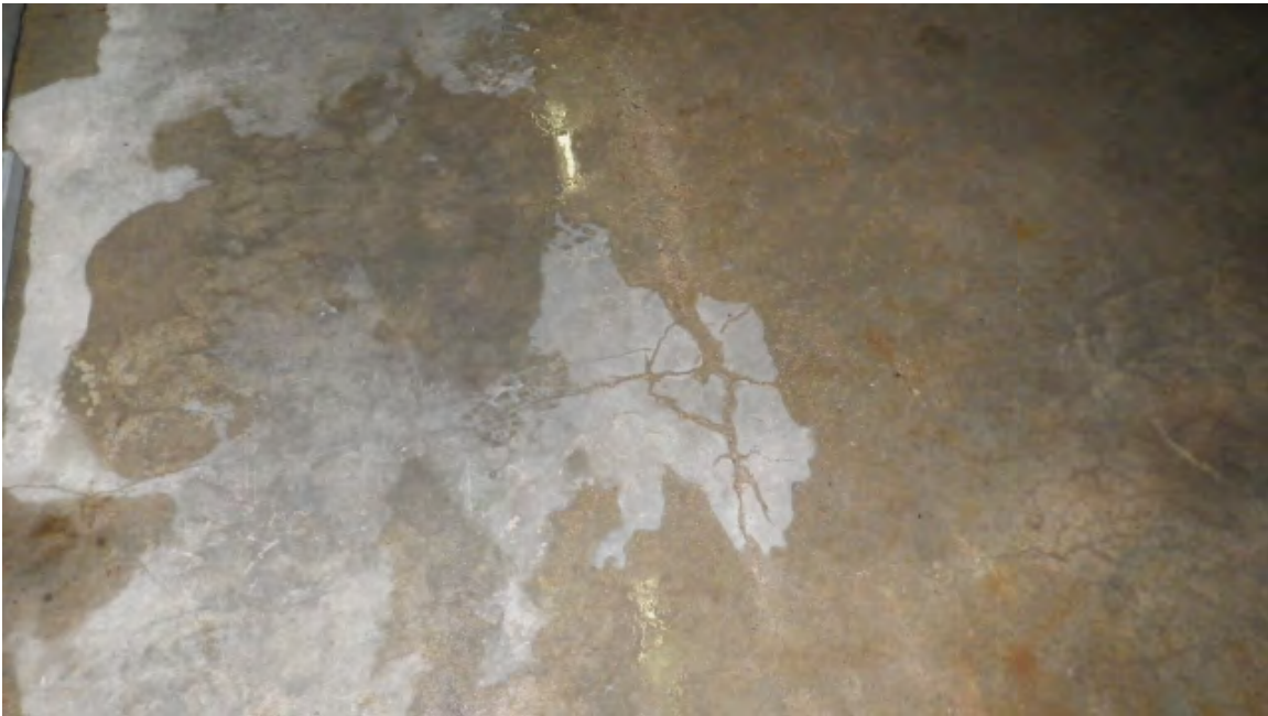
Photo 03 - Shrinkage cracking along Police Station slab on grade
