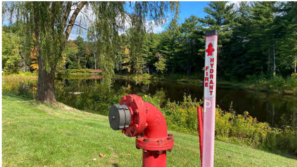
Hydrant for fire pond located along Beaver Brook Road.
