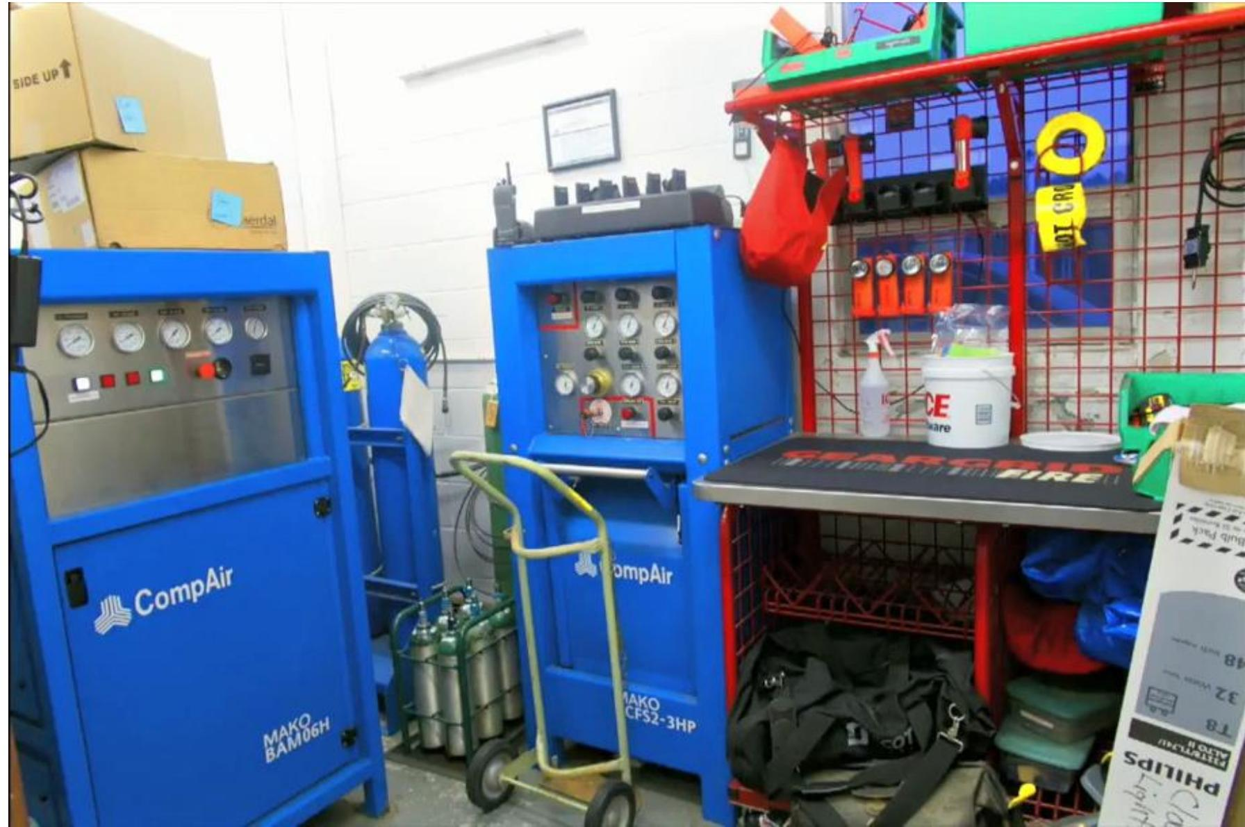
The critical self-contained breathing apparatus recharge equipment is not protected in a separate designated room, but stored in the radio service area and with the Boxborough Emergency Reserve Corps equipment
