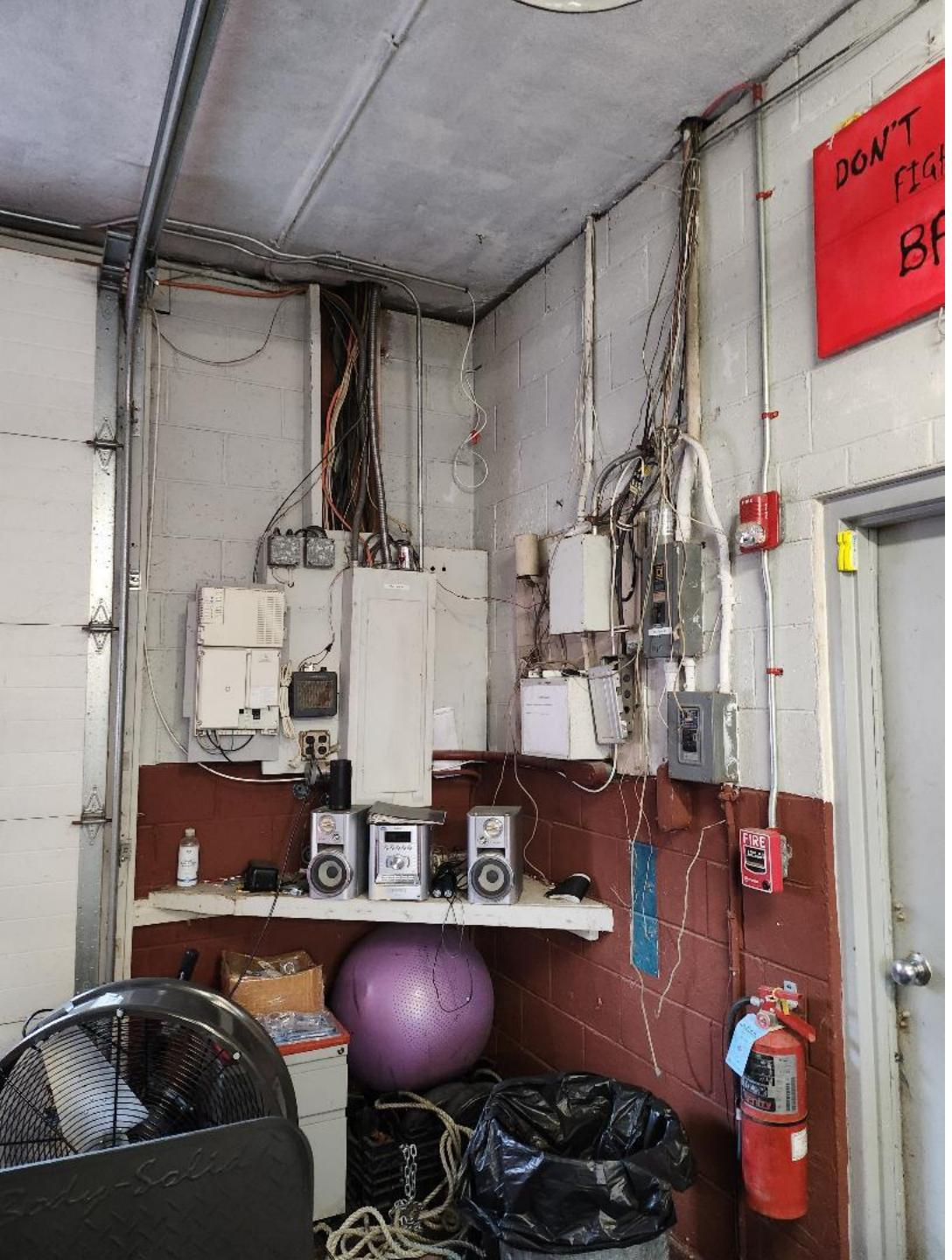
The firehouse main electrical panel sits in an open room with exposed cables, wiring and related equipment. The equipment is unsecured, with no electrical vault or cabinet
