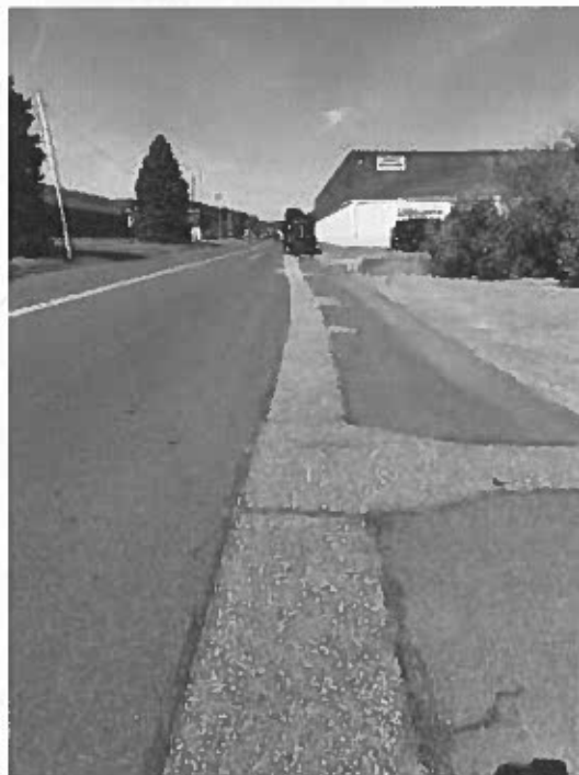
Trenching condition not acceptable. Straight trench cuts are required. Haphazard / inconsistency in sawcut & no joint sealer.
