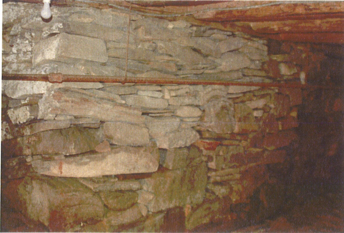
PHOTO #3 - Other Wall Supporting Chimney
