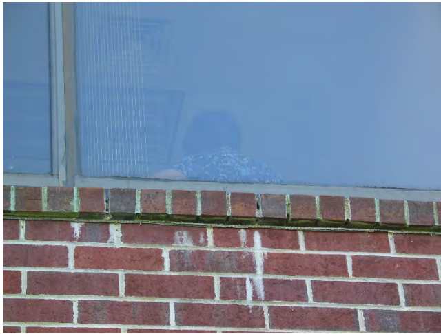
3 - Deteriorated mortar joints and efflorescence
