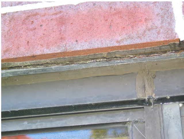
15 - Sealant installed above flexible flashing at the head of a window preventing water from exiting from wall cavity.
