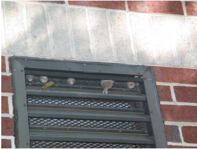
10 - Example of louver with no visible flashing or weeps at head
