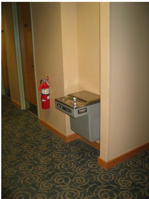
23 - Typical single level, non-ADA compliant drinking fountain outside toilet rooms.
