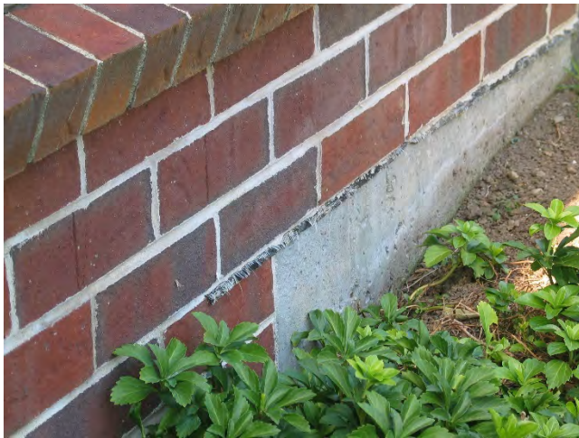
11 - Degraded flexible membrane thru-wall flashing where masonry meets concrete foundation wall
