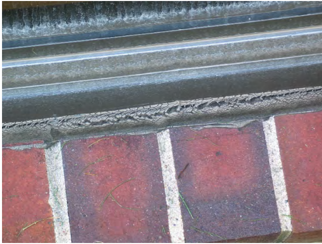
14 - Cracked and deteriorated sealant around windows.
