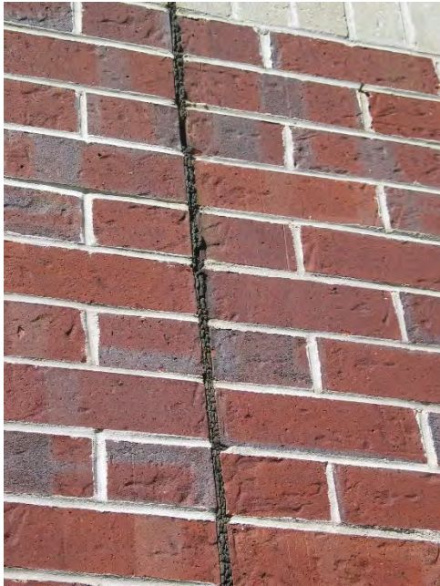
16 - Cracked and deteriorated sealant at masonry control joint.
