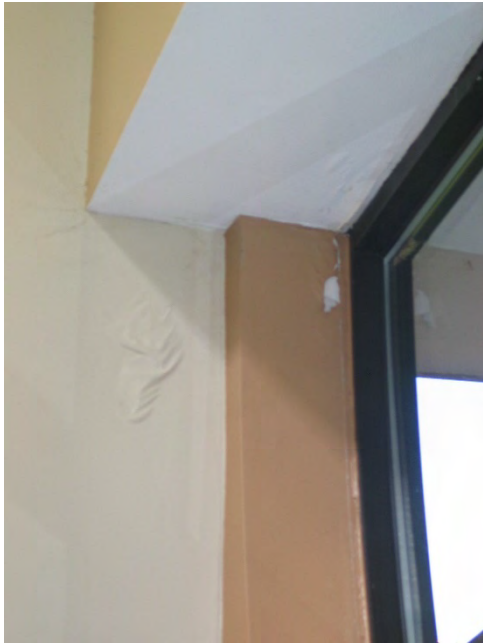
20 - Chipped and peeling paint from water intrusion at head of lobby storefront. Water penetration likely from storefront above at second floor level entrance canopy.
