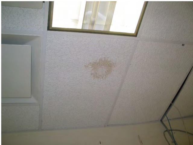
21 - Water stained ceiling tiles on the second floor.
