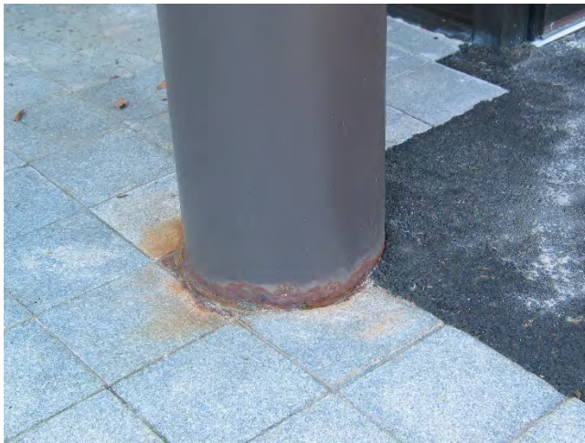
9 - Corroded column at main entrance canopy
