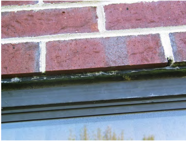
12 - Degraded flexible membrane thru-wall flashing at window head
