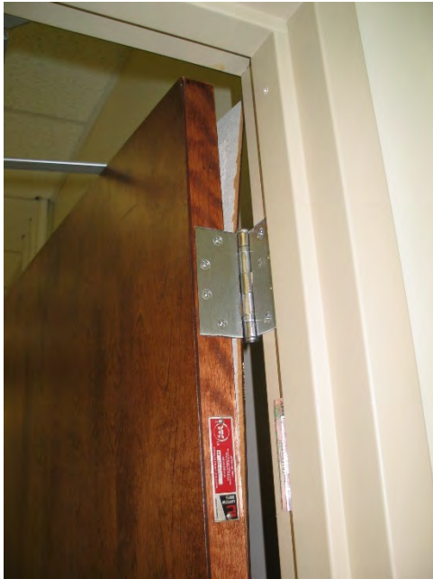
22 - Delaminating wood veneer at wood door in second floor tenant space.
