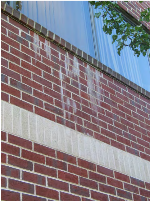
2 - Efflorescence below window sills
