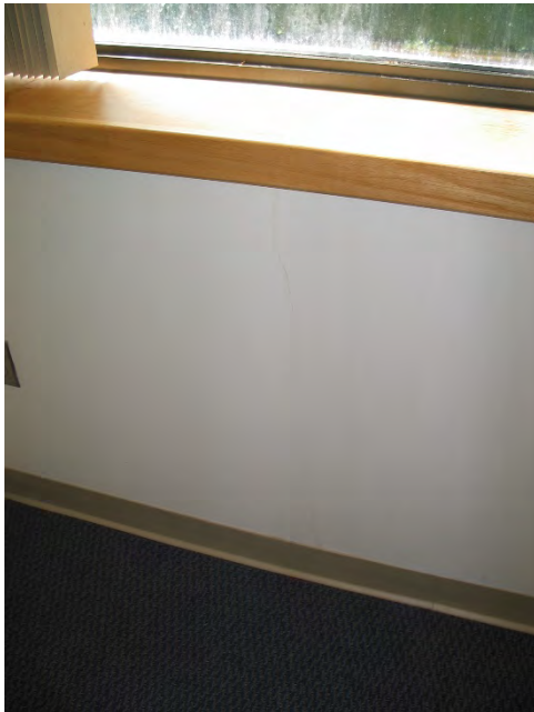
19 - Water stained drip running from under wood window sill down to wall base at second floor window along west wall.
