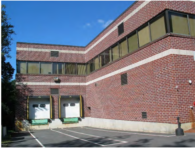
28 - Opening at the first floor in the corner is location of door exiting from egress stair. Note the close proximity to the truck loading bay. A vehicle in this location could impede emergency egress.
