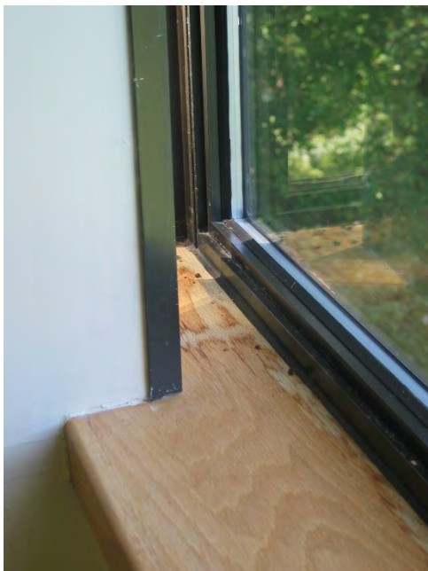
17 - Water stained wood window sill at second floor window along north wall.
