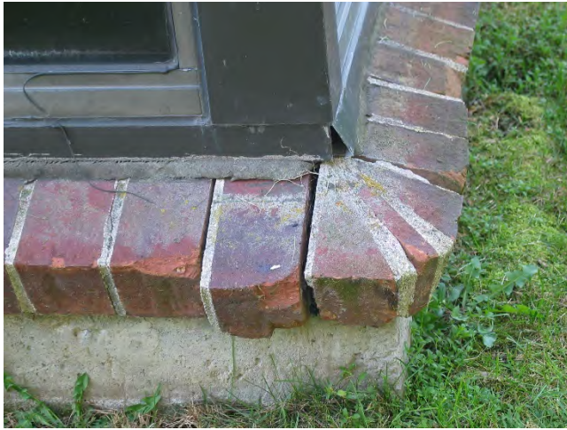
4 - Brick window sill requiring repointing
