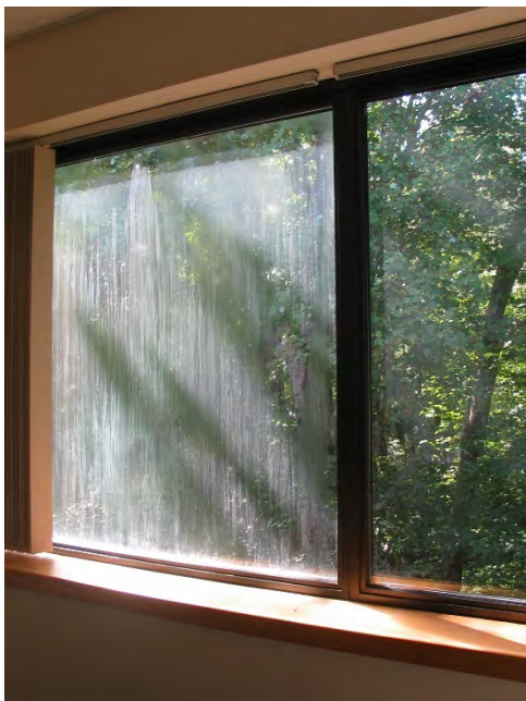
7 - Etched/fogged glass indicative of failed window seals
