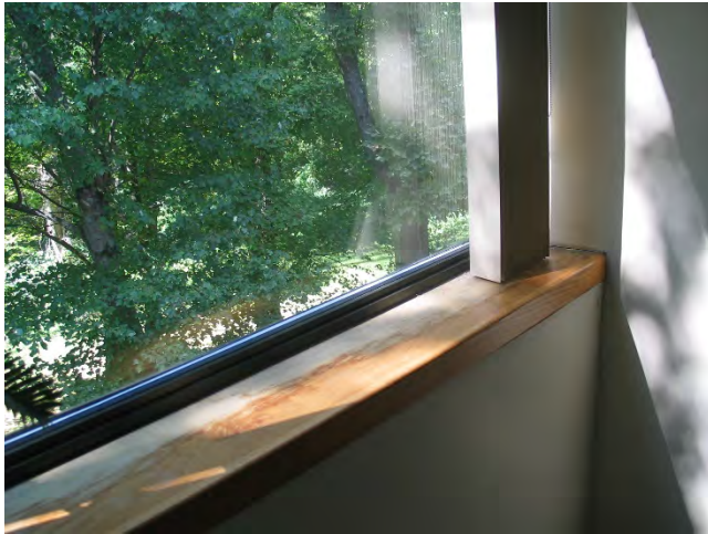
18 - Water stained wood window sill at first floor window along west wall.
