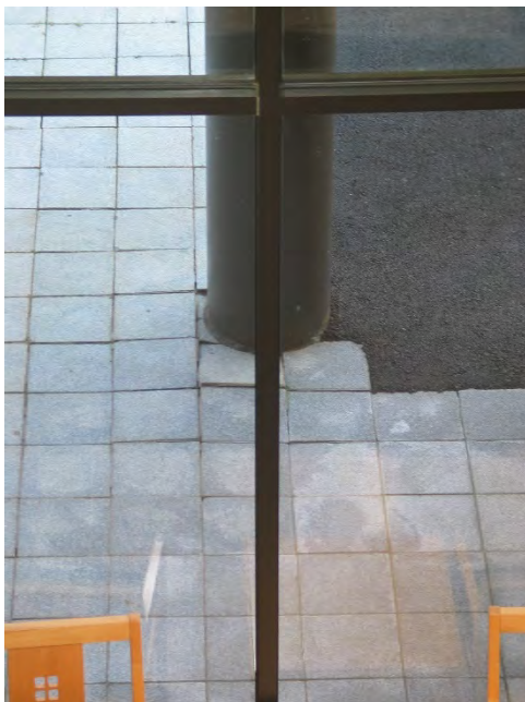
25 - Pavers at main entrance provide an uneven walking surface.
