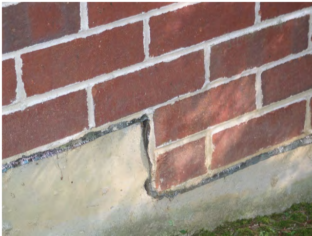
13 – Improperly installed flexible membrane thru-wall flashing at stepped foundation wall. No end dams are visible.
