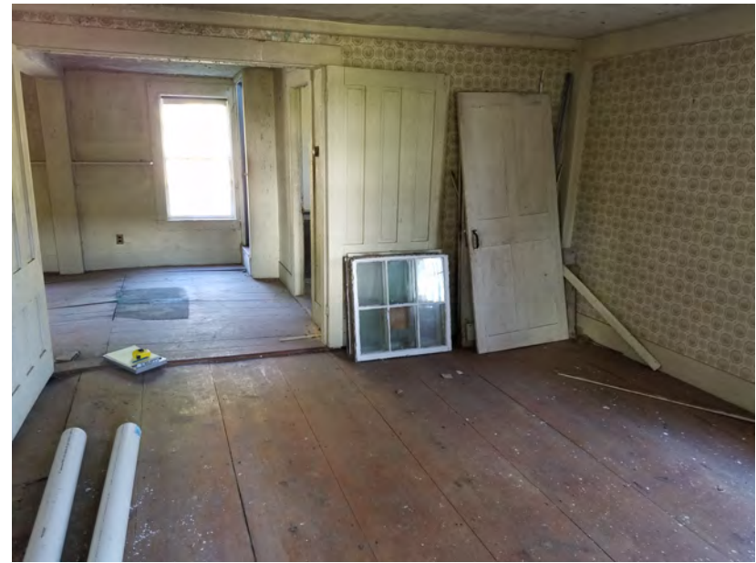
Historical sash stored in the house
