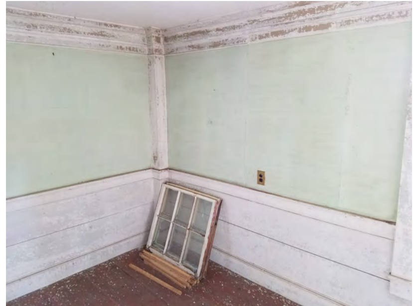
Wainscot and cornice at the East Chamber, floor 2.
